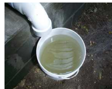
Dirty first-flush water
